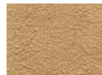
LEAVES CONCRETE LOOKING LIKE NEW AFTER GRAFFITI REMOVAL
